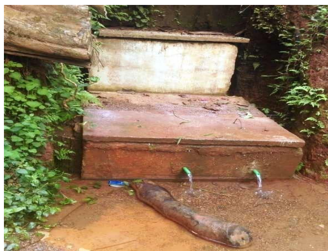
Plate 4.1. Plate indicating an improvised water collection point (Photograph; 17/ 09/ 2020)
